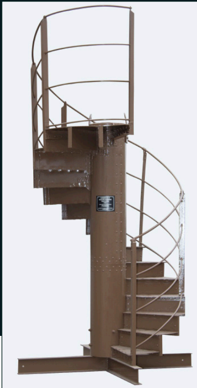
Gustave EIFFEL Staircase from the Eiffel Tower n° 17 - 1889 In bolted wrought iron
